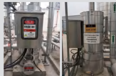
提供给韩国三星EP级电子气水浴式气化器 Electronics Gas Project for Samsung, EP grade Water-bath vaporizer
