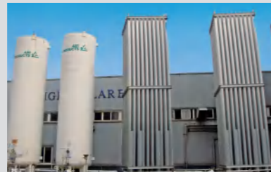
Air Products空温式气化器现场 Jobsite of Air Products Ambient Vaporizer
