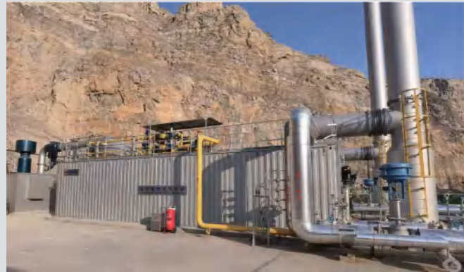
为济南能源集团提供2台浸没燃烧式气化器现场 Jobsite of 2 sets SCV for Jinan Energy Group
